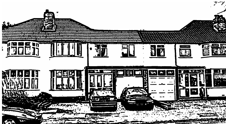
✗ Terracing effect and loss of gap between properties originally built as semi-detached
